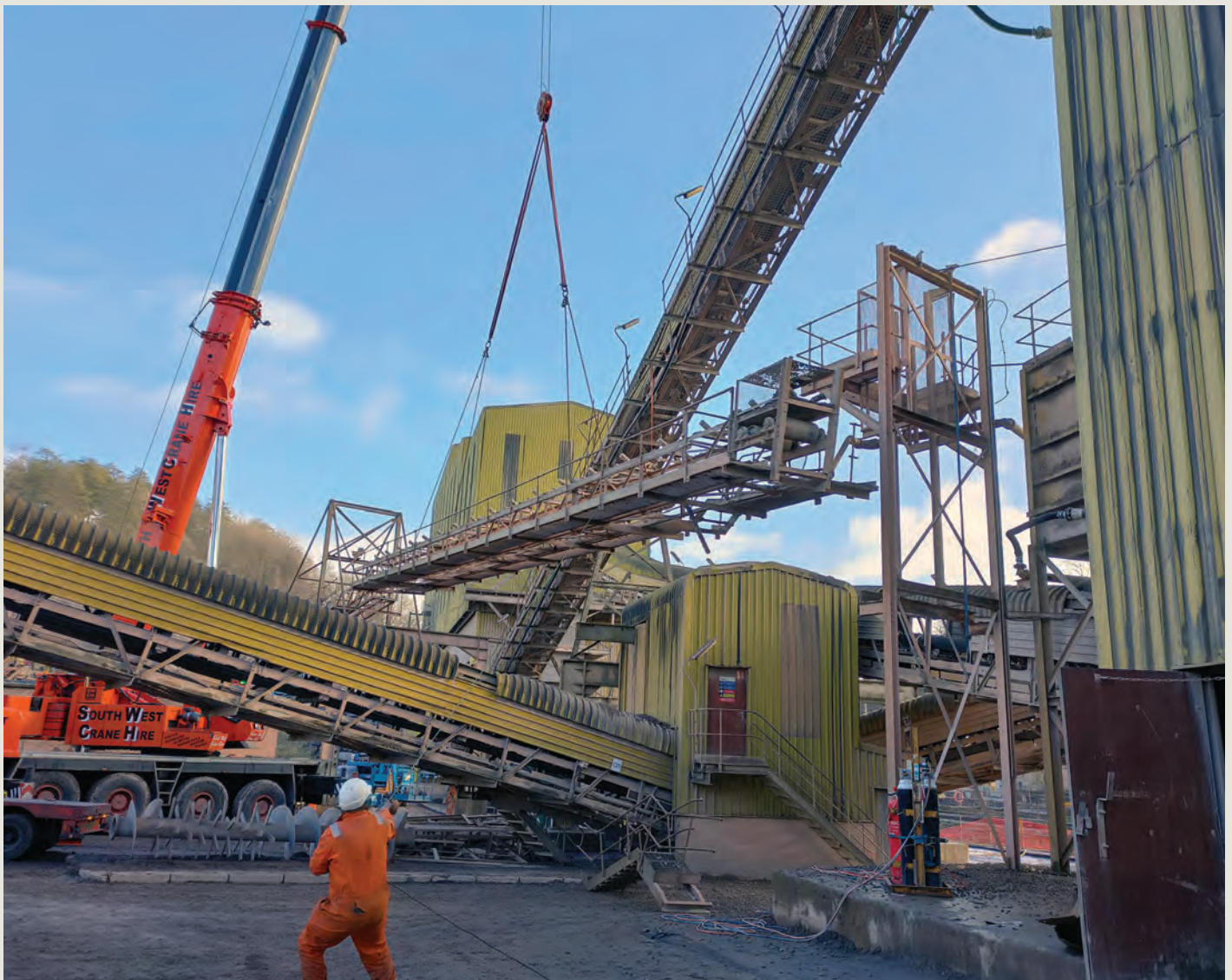
Above: the new crusher at Whatley Below: a crane repositions a conveyor belt as part of the quarry revamp
