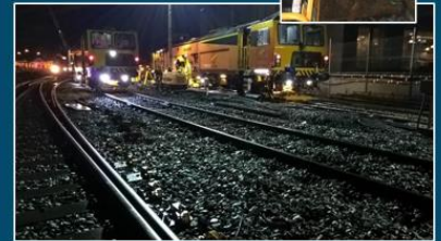
9. Consolidating track stone
