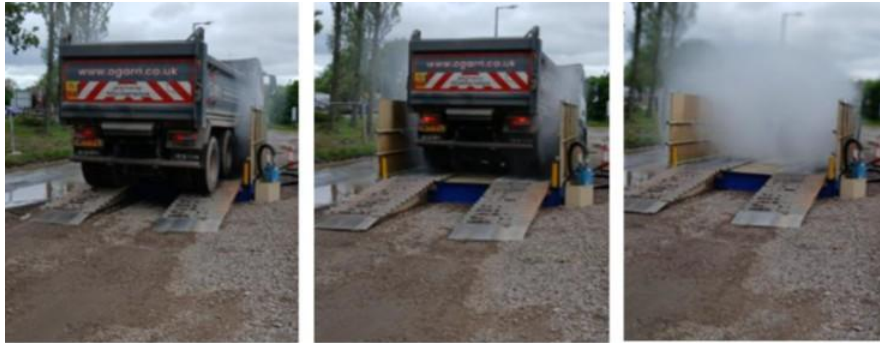
Construction Site Wheel Wash in Operation
