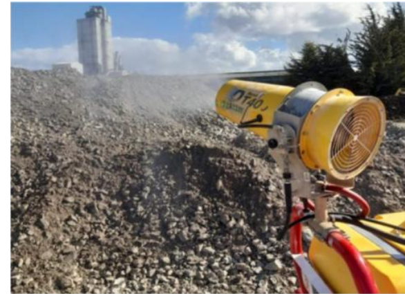
Mobile Mist Spray Cannon in Operation (Dampening Down Stockpile)
