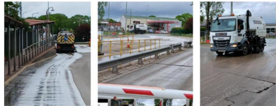
Plant Road Sweeper / Water Dust Suppression In Operation
